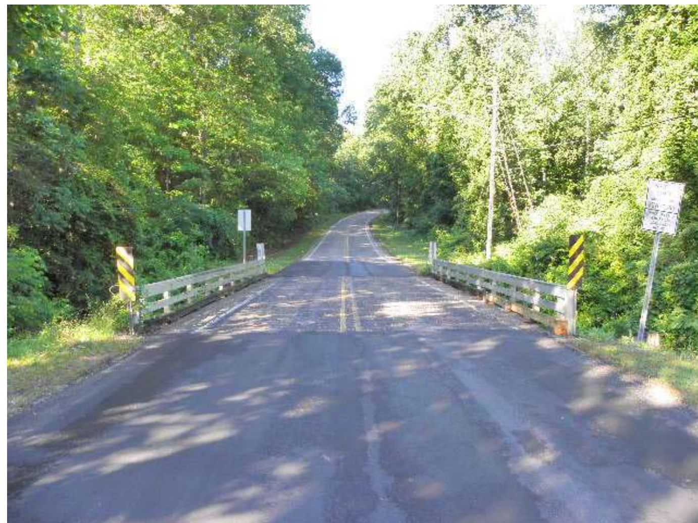
View Facing South (Downstation)
