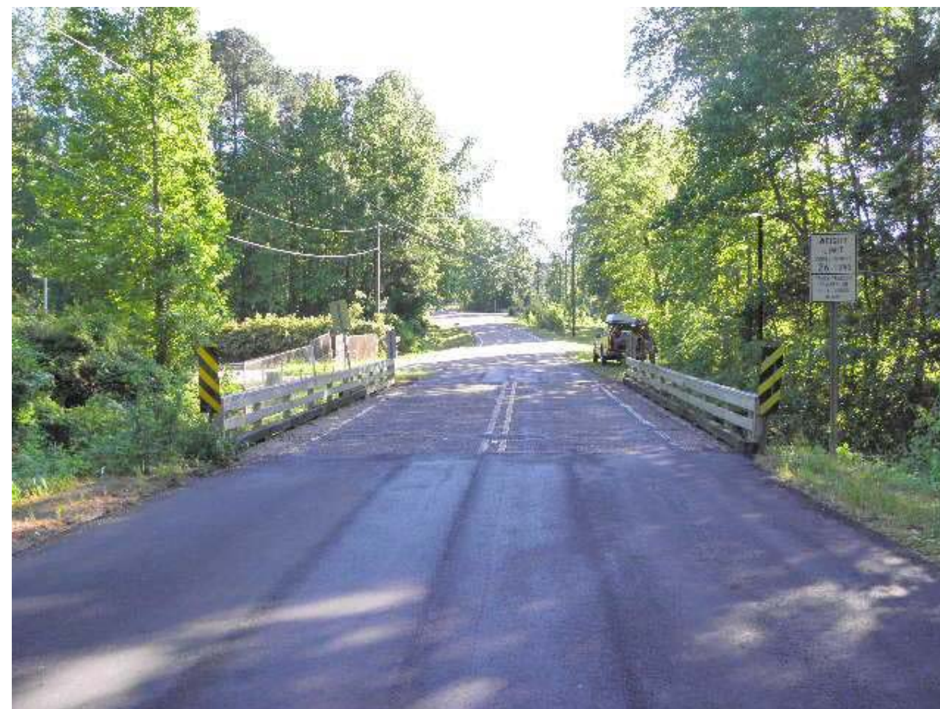
View Facing North (Upstation)
